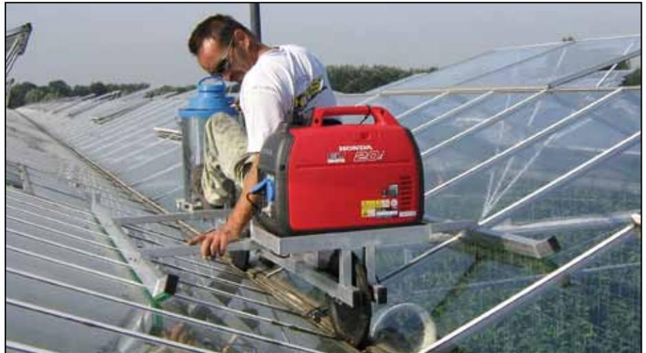
Image 1: Use of the "roof bicycle" to inspect the glasshouse roof and clean the gutters
